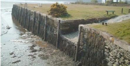
This highlights an important safety issue of the current design, as small craft have to be lifted from the water up to the level of the current slip, should the time of high water be missed. At present, in order to launch any marine craft a tidal height of 4.7m is required. This equates to only 27 hours over a two-week period (under 2 hours per day). An extension to the slipway is proposed, which would lengthen the
